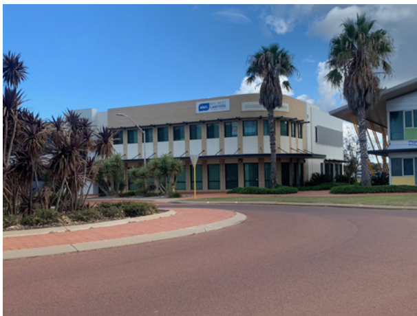
The new YSRC offices on Wiebbe Hayes Lane in Geraldton.
